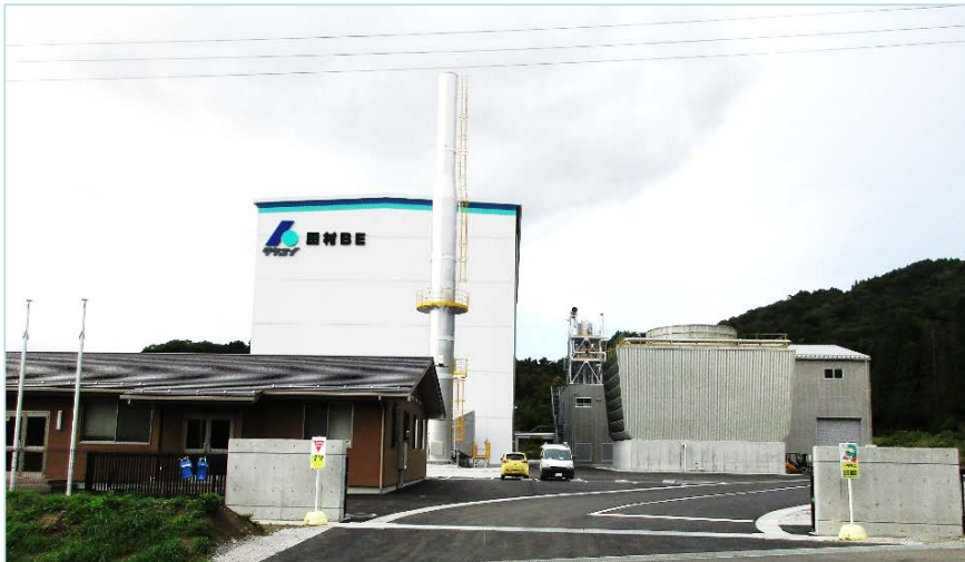
The new plant will be named 'Tamura Biomass Power Generation Plant'.
