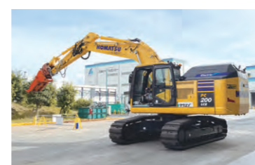
The excavator trialed at TAKEEI's Kawasaki Recycling Center
