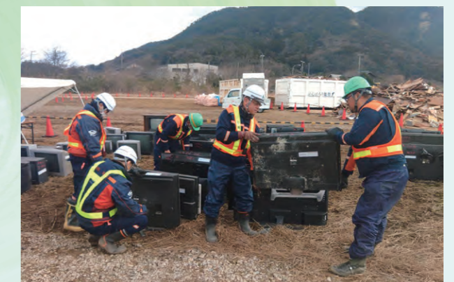
The temporary waste storage site
